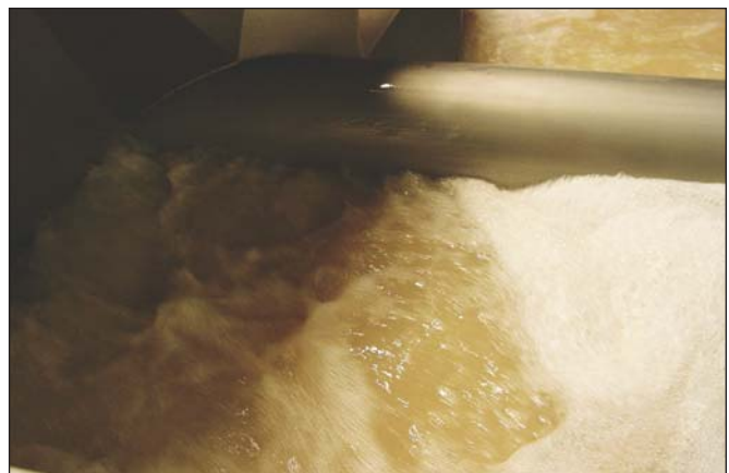
Chiller after adding Spectrum™
